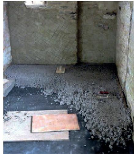
*A limecrete slab being laid over a geotextile separation layer with clay aggregate below: the result is a solid floor that 'breathes' across its entire surface. (Photo: David Blair)*
